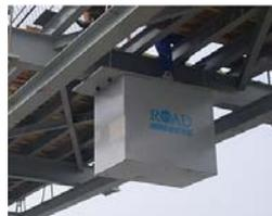
Figure 2. The TMD used in the passenger foot-bridge (taken from <http://www.roadjz.com/en/show.asp?id=18>)
